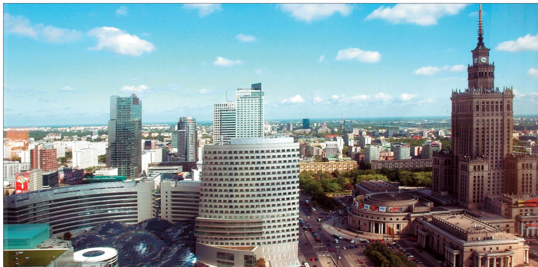
Old and new side-by-side: aerial view of Warsaw's Golden Terraces (Zlote Tarasy) and Palace of Culture and Science
