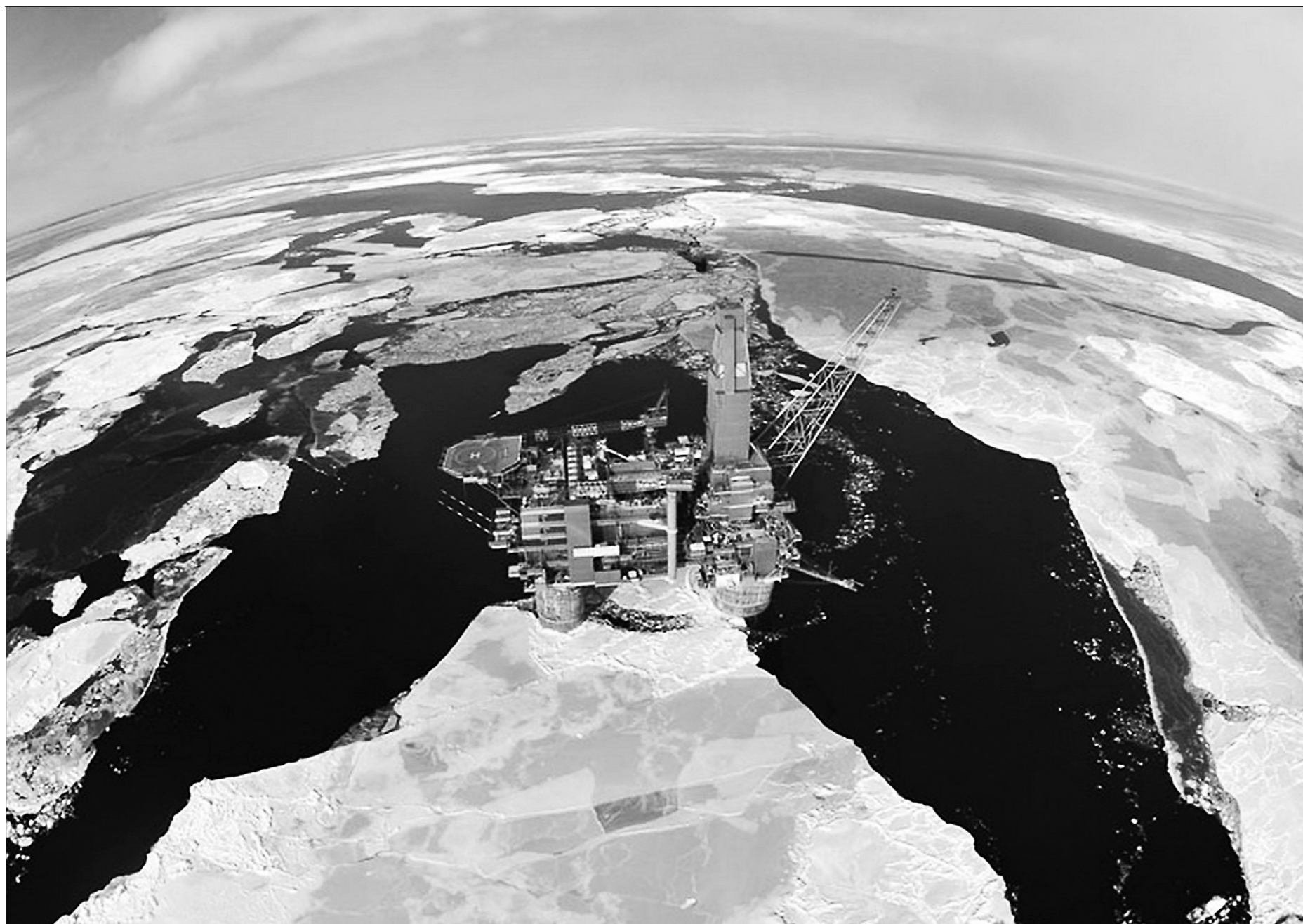
Russia's first offshore gas development: the Sakhalin II oil and gas project in the sub-Arctic Sea of Okhotsk has a huge liquefied natural gas plant
