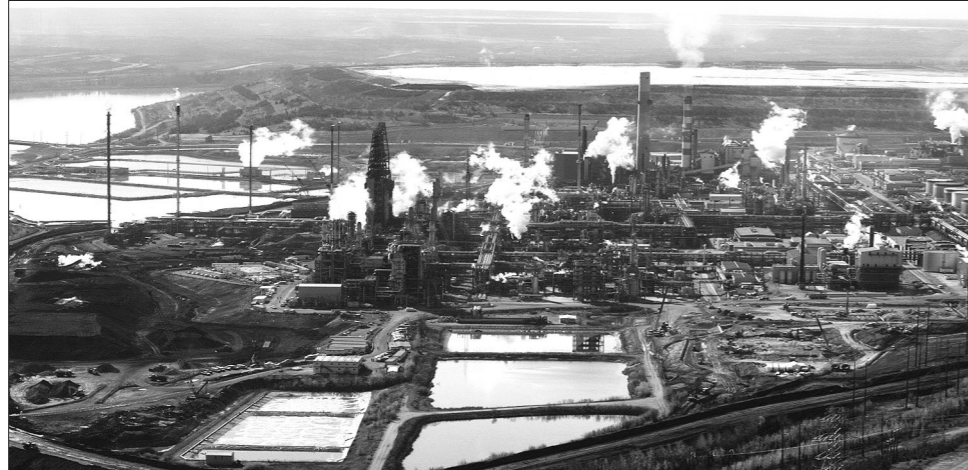
Plant at Fort McMurray in Alberta, the centre of the oil sands industry
