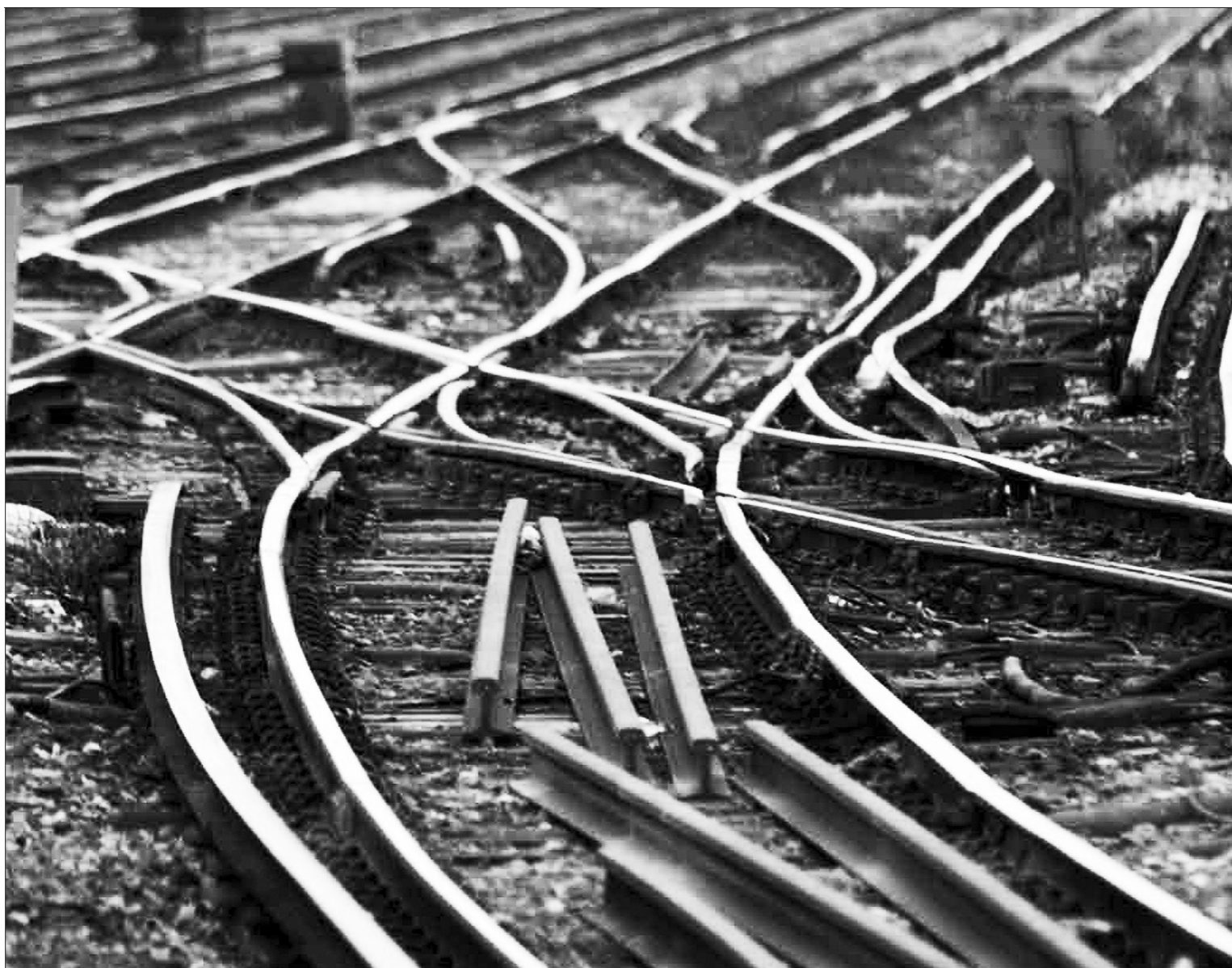
To the point: network operators aim to replace equipment just before it fails, rather than long before – or just after
