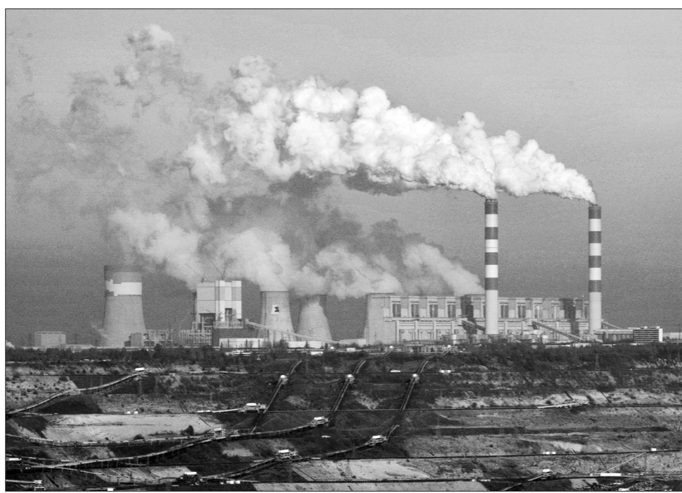
Crisis generation; water vapour and smoke rise from a power station in Belchatow Bloomberg
