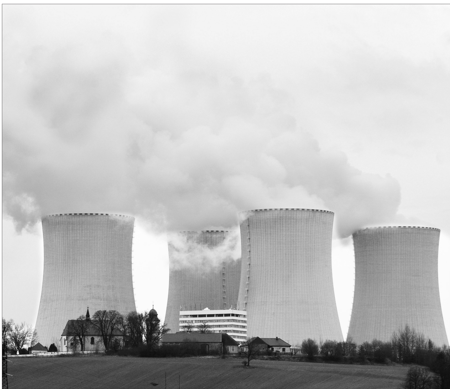
Steaming ahead: vapour rises from the cooling towers at the Temelin nuclear power plant. In October, a project to build two reactors begins in earnest
