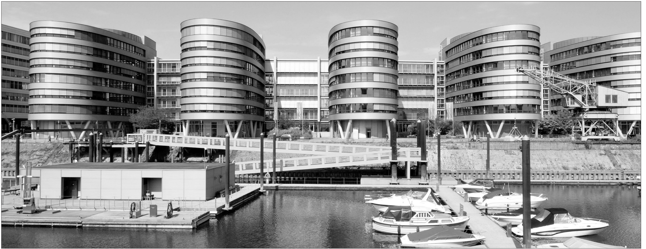
Redevelopment of the harbour area has lured businesses, tourists and residents with a mix of offices, museums, shops and restaurants
