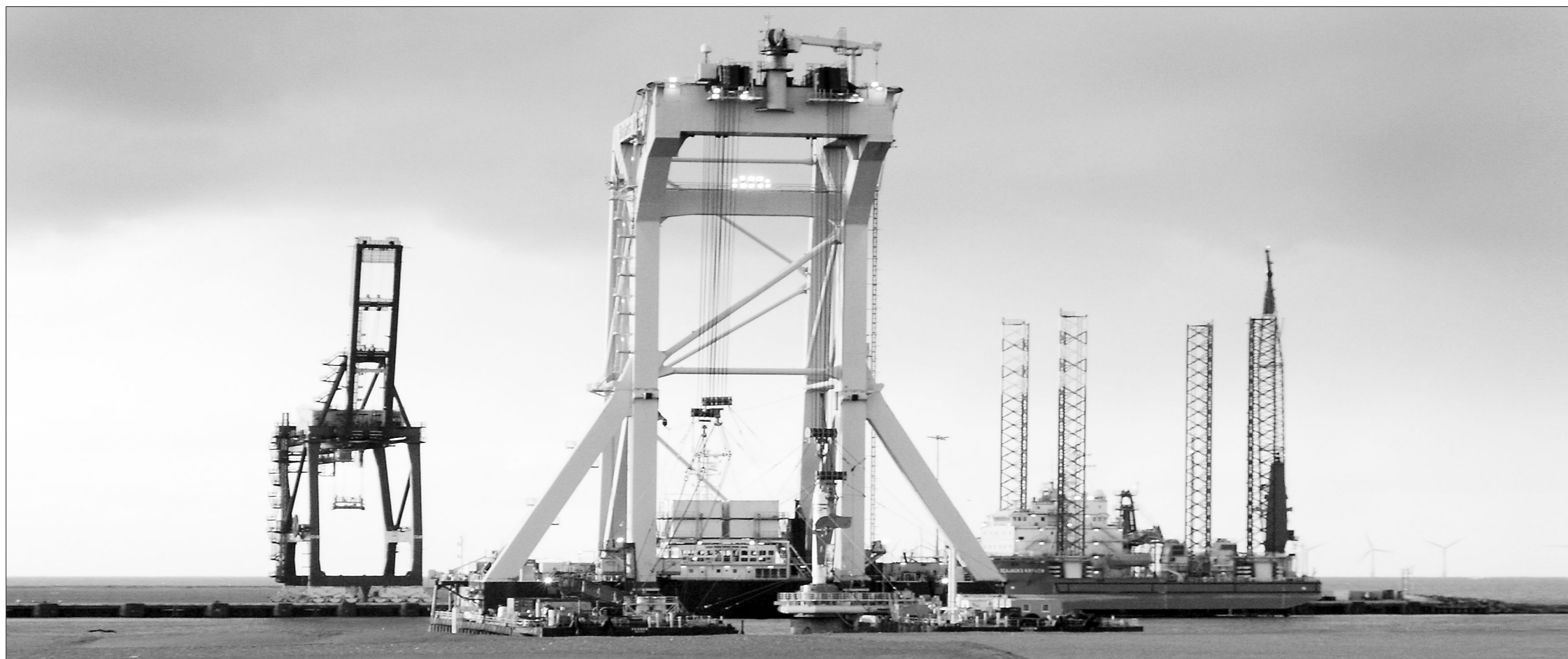
Quay point: the Seajack Kraken barge at Great Yarmouth's expanded port
