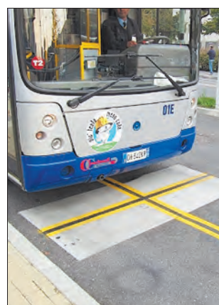
Grid locked: battery charger
