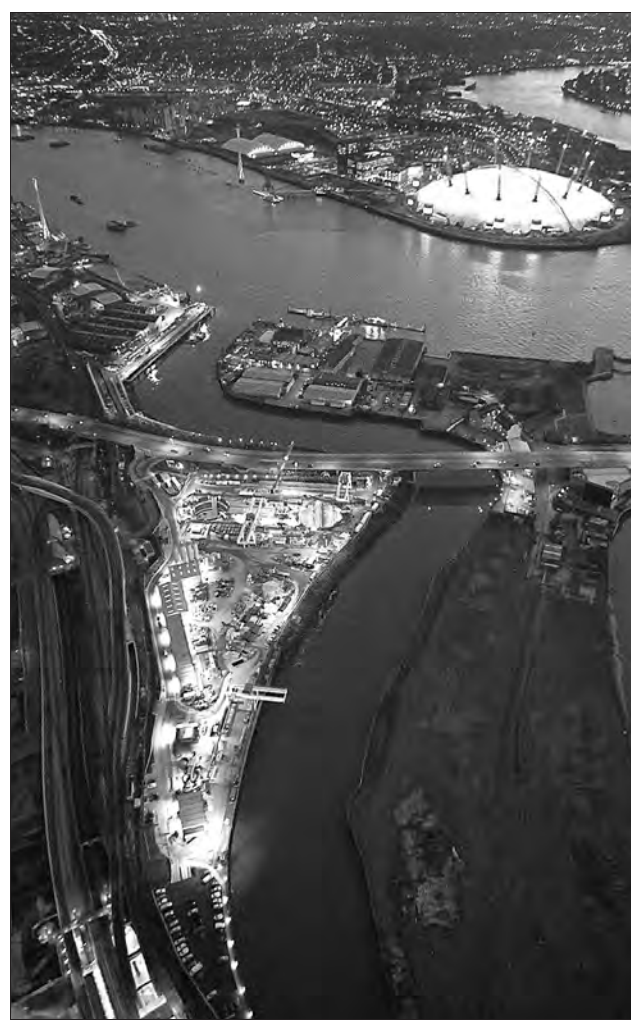
Eastern approach: the Crossrail construction site at Canning Town
