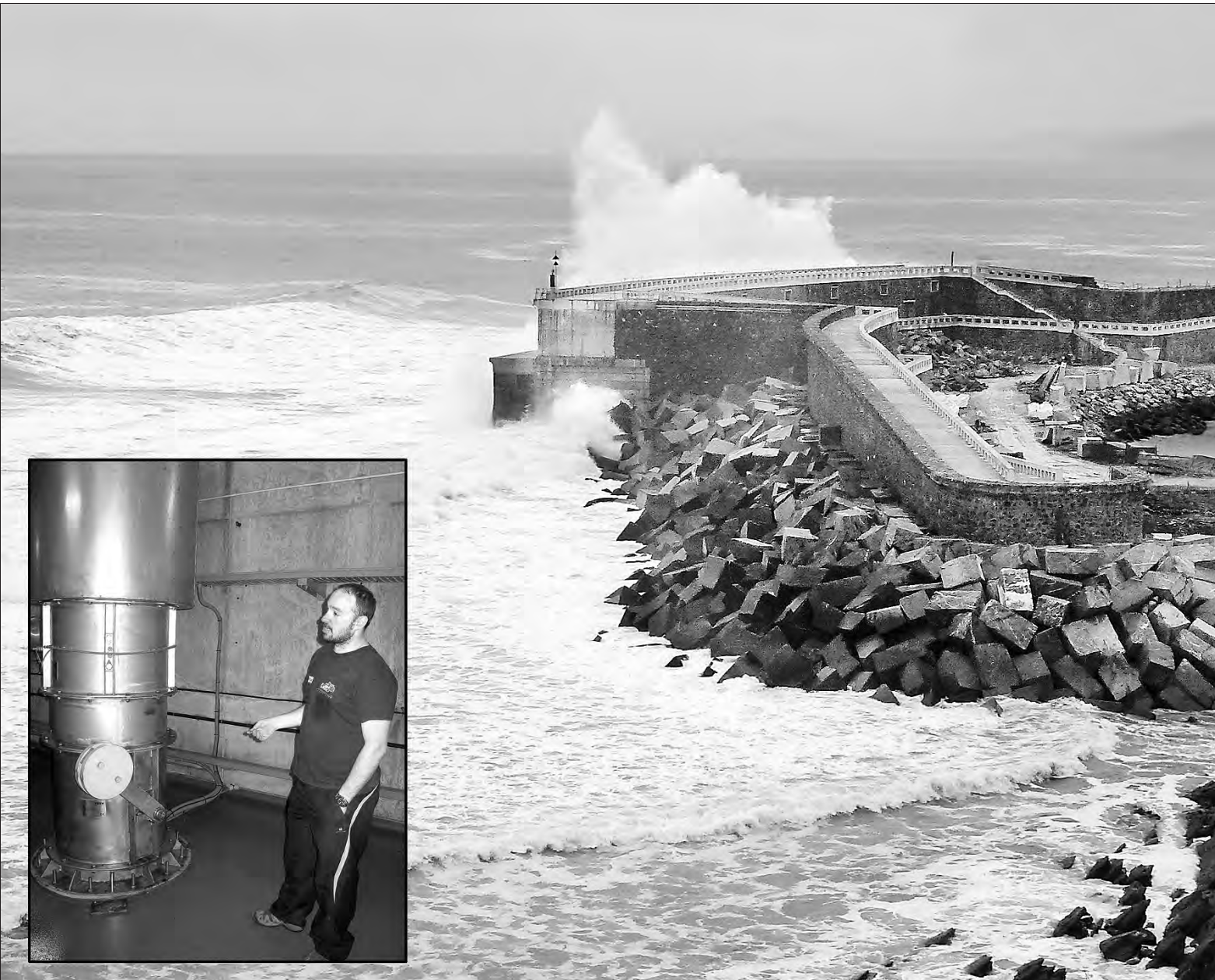
Making waves: interior and exterior of the Mutriku plant, which uses 'oscillating water columns' technology
